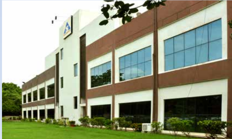
Sanmar Engineering, Karapakkam.
