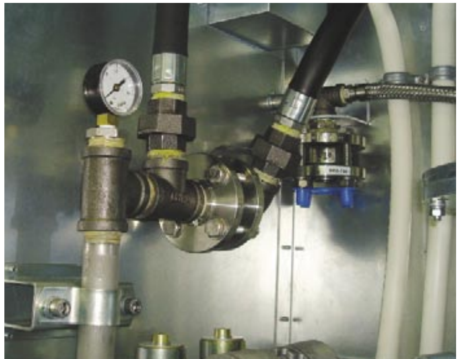
Rupture disk assembly in Bloom Box.
