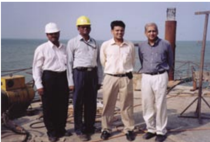
Vijay Sankar seen inspecting the construction of the marine terminal facility at Karaikal along with V Ranganathan, Chief Executive S Venkatesan, GM - Operations and Veludas, Site Engineer, Fichtner Consultants.
