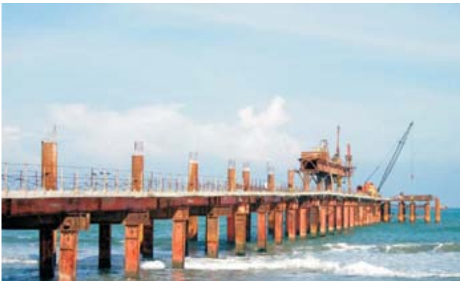
Work on Marine Terminal Facility in progress on the seafront.
